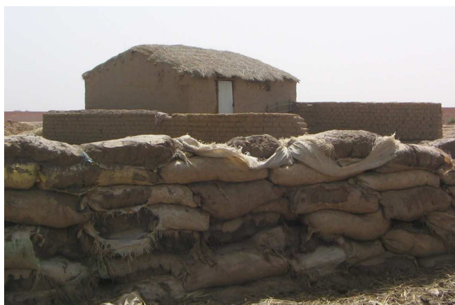
Figure 53: Mur de sac de banco (Bargodaga/Mopti)
